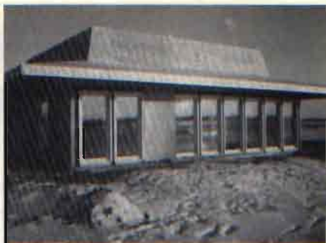
STEINBACH FLY-IN CLUB'S new clubhouse under construction
