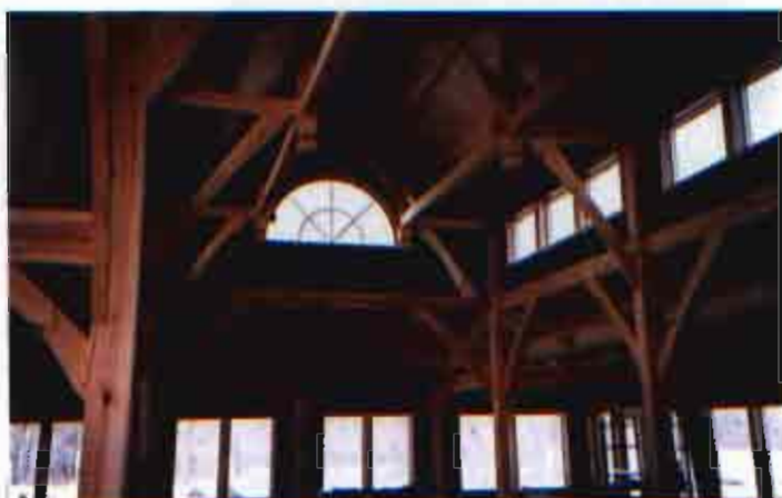
Timber-frame construction is featured in new clubhouse to open in mid-May at the Bridges Golf Course.
