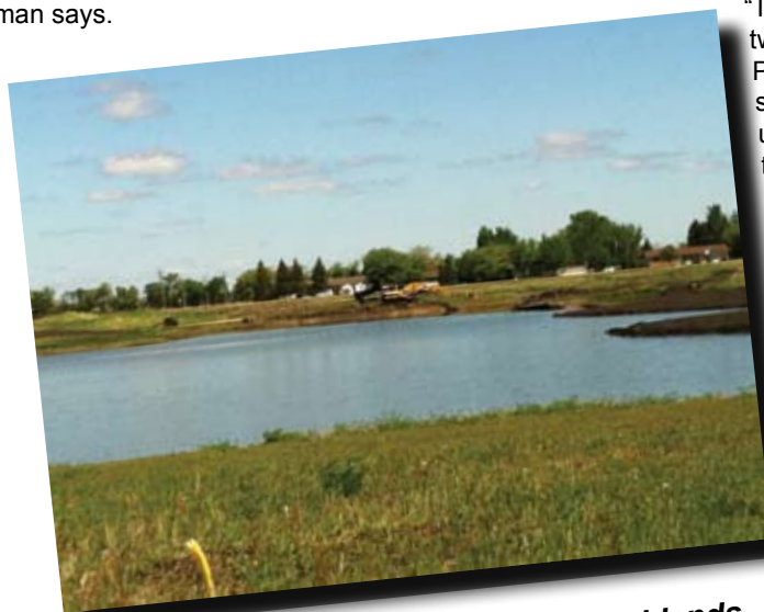
Work is in progress at The Highlands.
